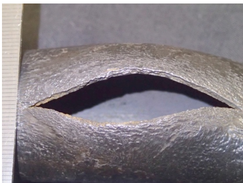
Fig. 6. TO 2, damaged pipe
